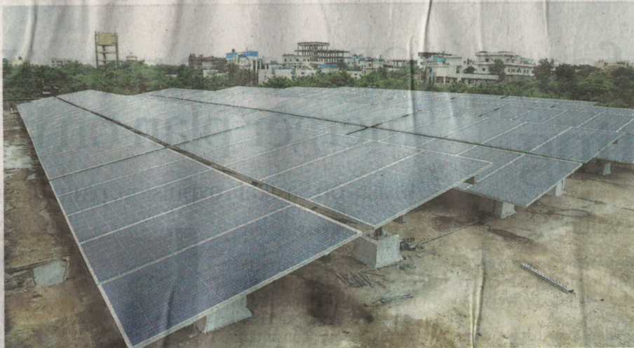
Energy-efficient: The 396.8 kWp rooftop solar plant set up on one of the buildings at ESSO-INCOIS, Hyderabad. • BY ARRANGEMENT
