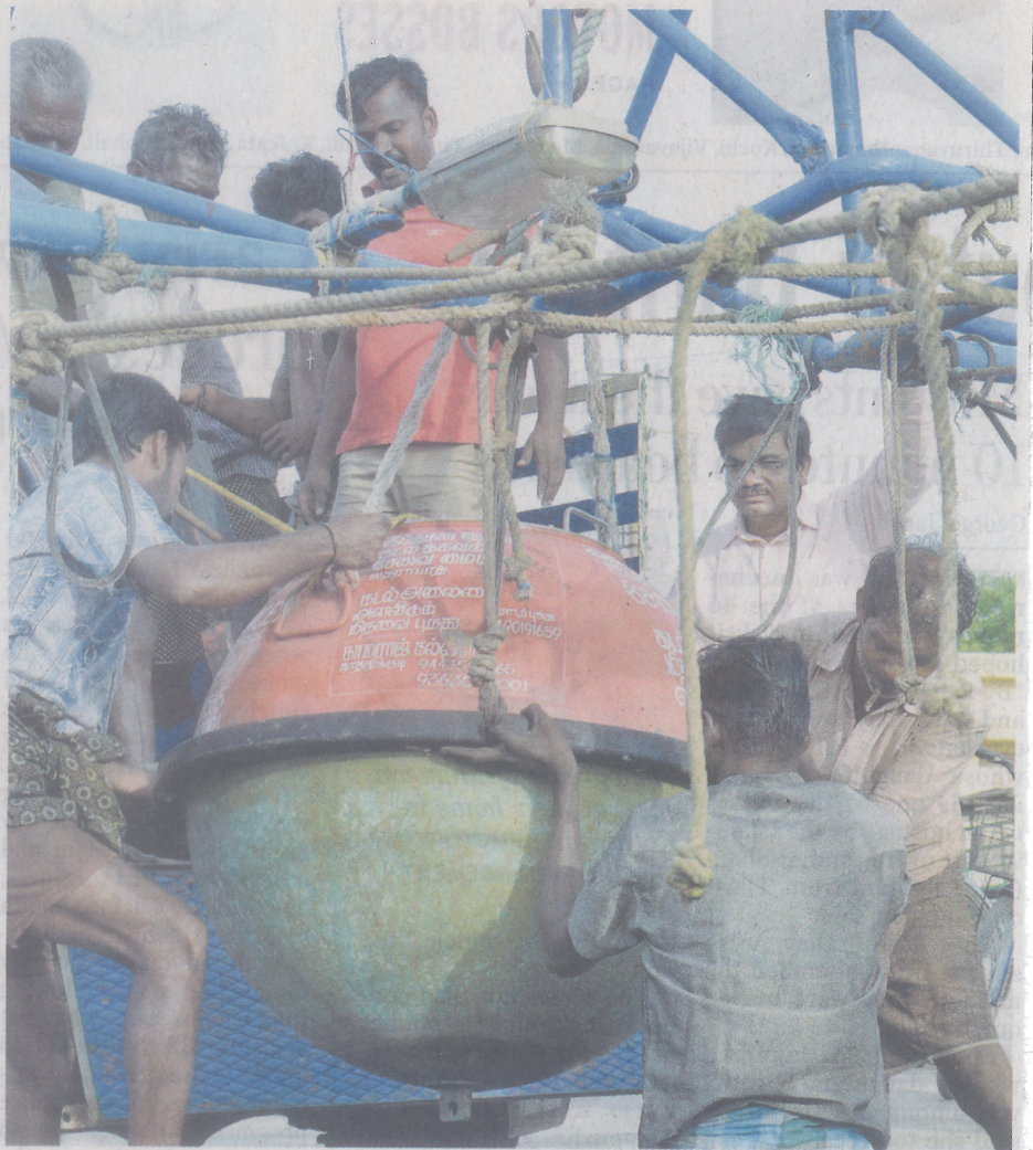
IN PLACE: A wave rider buoy being installed in the waters on Tuticorin coast on Thursday. – PHOTO: N. RAJESH
